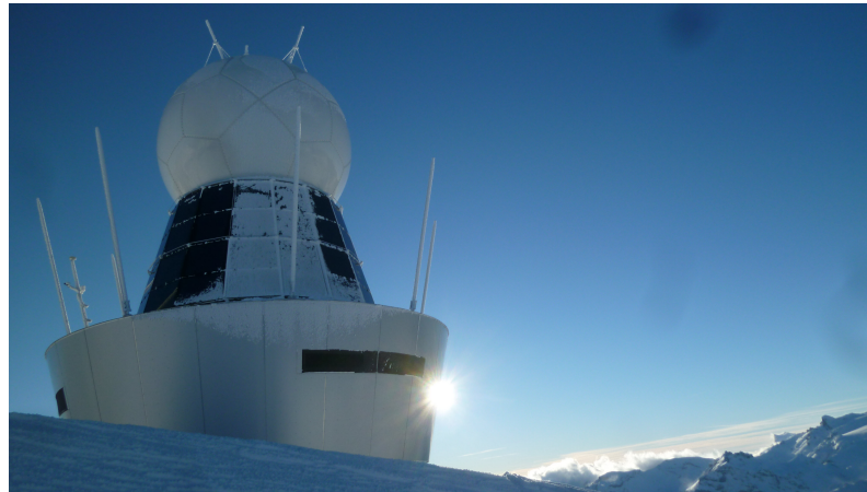
Figure 13. Picture of the radar on Pointe de la Plaine Morte, 2937 m above sea level. The lightning protection consists of two groups of lightning poles, one below the lowest point of the antenna, and the other one on top of the radome. This design results in minimal interference of the lightning poles on the radar beam and polarimetric measurements.
