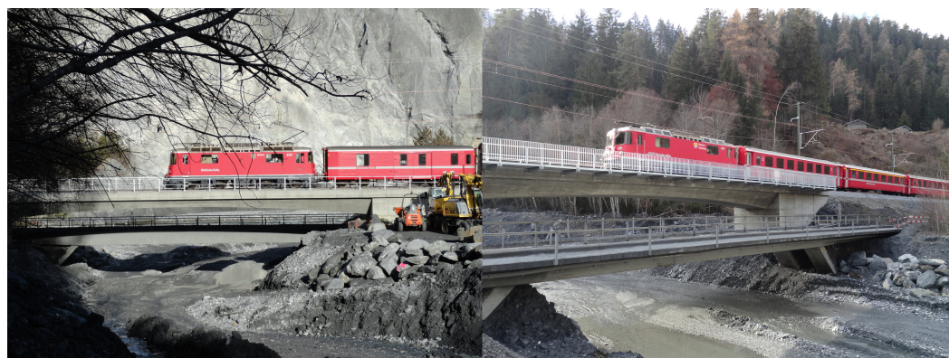
Figure 6. Inauguration of a new railway bridge in the Grison Alps in eastern Switzerland in 2011. The new bridge is three metres higher than the old one and was built to protect the rails from increasing threats of flash floods and debris flows. A customised radar-based heavy precipitation warning system was put into operation on 7 August 2017. One day later, the nowcasting system issued its first warning, and a few minutes later the rails on the new bridge were flooded by a debris flow. Photograph courtesy of the Rhaetian Railway.
