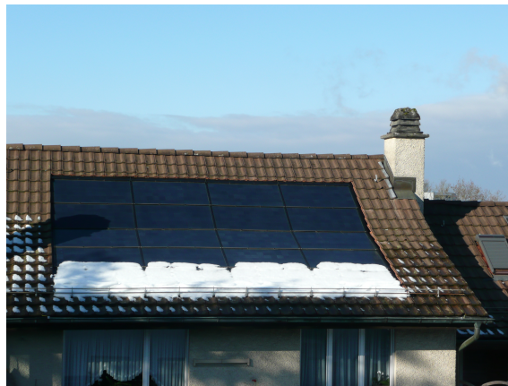
Figure 6: Example for a partly snow-covered PV panel leading to a reduction of the irradiated area and thus probably of the power production. Zurich, December 2013.
