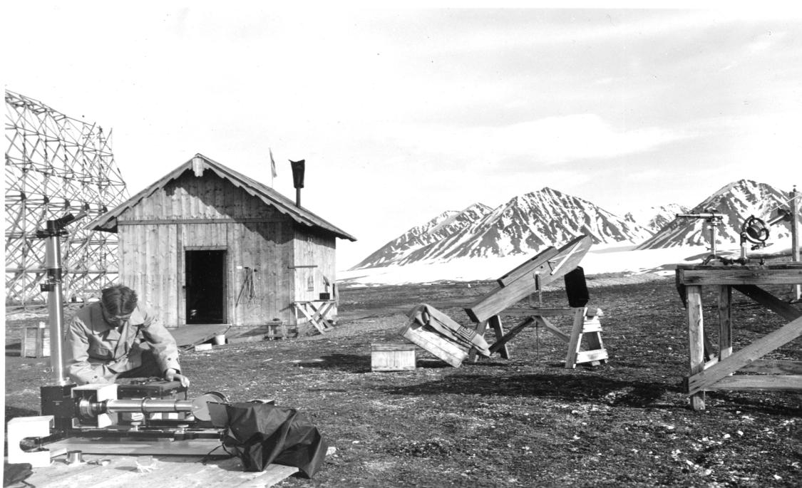
**Figure 19:** Cabin and instruments used by Götz during his measurements at Svalbard. Götz is adjusting the Arosa (Fabry-Buisson type) spectrograph. The Féry spectrograph is in the center. The instruments on the shelf (right hand side) are a Michelson actinometer (left) and a silver disk pyrheliometer (right). (Photo LKO Archives).
