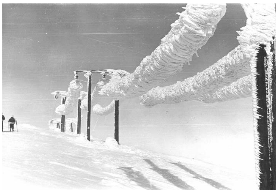
Figure A. 5 In-cloud icing on a 22 kV line feeding a TV tower 1 400 m above sea level in south-western Norway. (Photo: O. Wist)
