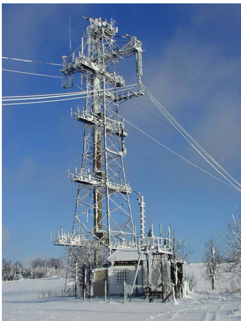
Figure A. 10 Test site at Studnice (Photo: J. Sabata)
