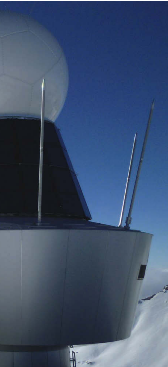
The radar on Pointe de la Plaine Morte, 2,937m above sea level after commissioning in November 2013. This is one of the two additional radar sites built to improve radar coverage in the Alps
